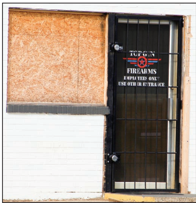
Top Gun Firearms was the target of property damage last week, though nothing was taken from the store, according to the Blairsville Police Department. Photo by Shawn Jarrard
